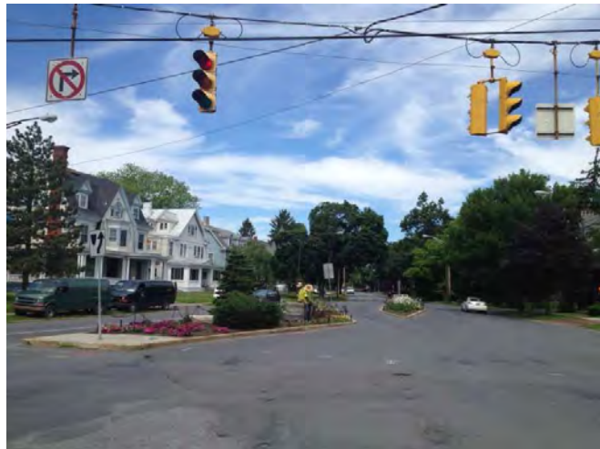
Complex intersection at Madison Ave and Western Ave
